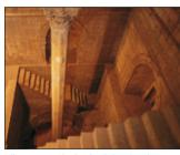
Nilometer on Rhoda Island showing the simple calibration used to predict the floods
