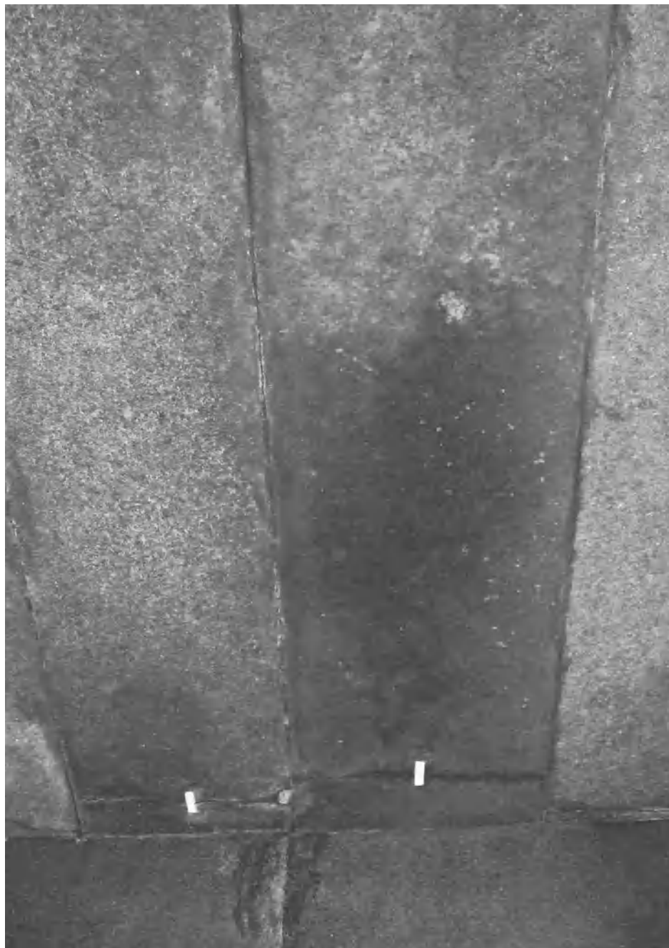
Plaster strips on the cracks in the King's Chamber help Egyptologists detect if the cracks get larger.
