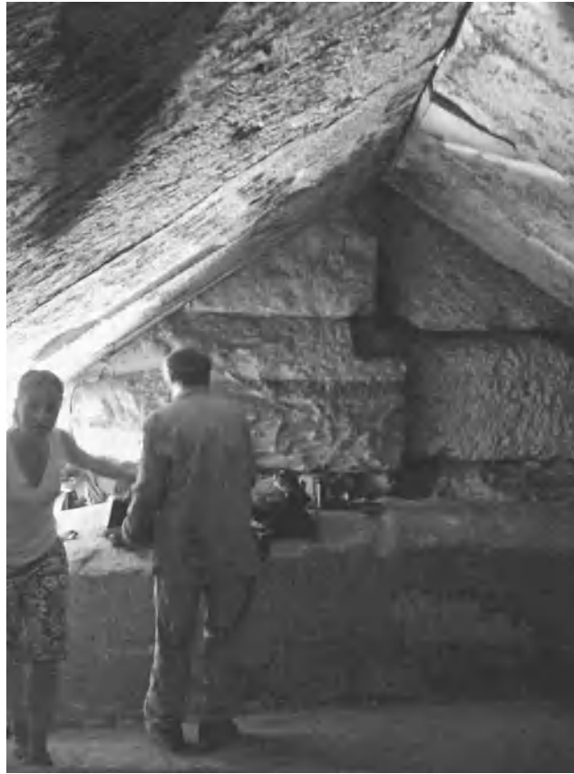
Above the last relieving chamber are huge limestone rafters to take the weight above off the ceiling below.
