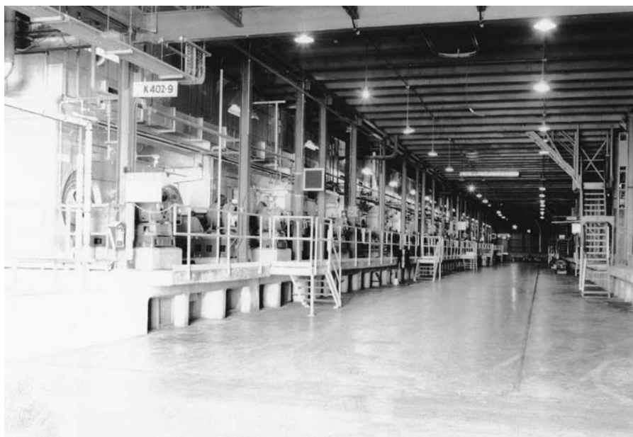
uranium isotope separation The huge K-25 complex at Oak Ridge, Tennessee, used a gaseous diffusion method to separate uranium 235 from the more plentiful uranium 238. Part of the facility, long abandoned because of radioactive contamination, is shown here during clean-up. U.S. Department of Energy
