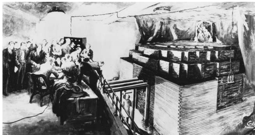
nuclear reactor Enrico Fermi can be credited with building the first successful nuclear reactor, Chicago Pile-1, at the University of Chicago in 1942.
