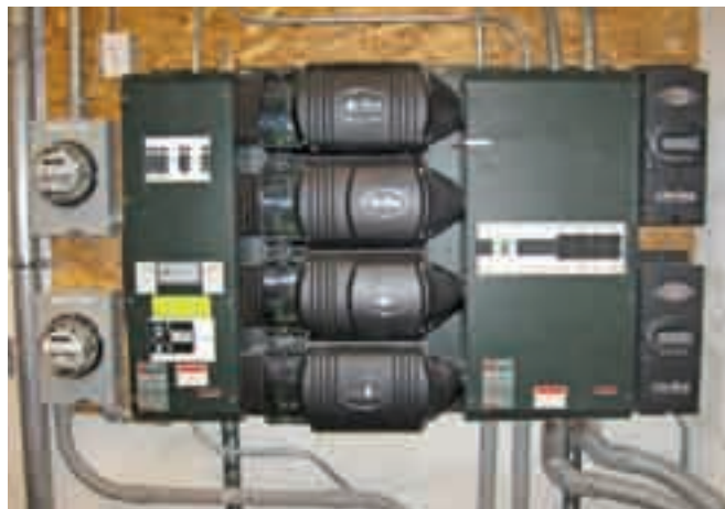
This large home system uses four OutBack charger/inverters in a 120/240 output configuration. The middle two inverters are mainly used to achieve a C/13 charge rate for 2,200 Ah of batteries at 48 V.
