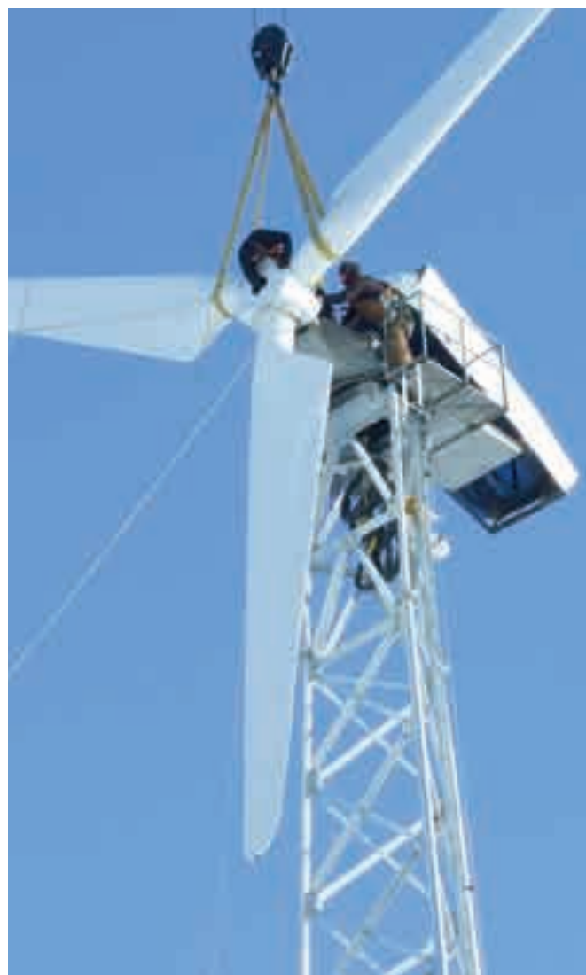
A Vestas V-15 rotor being installed on the turbine by a crew of four.
