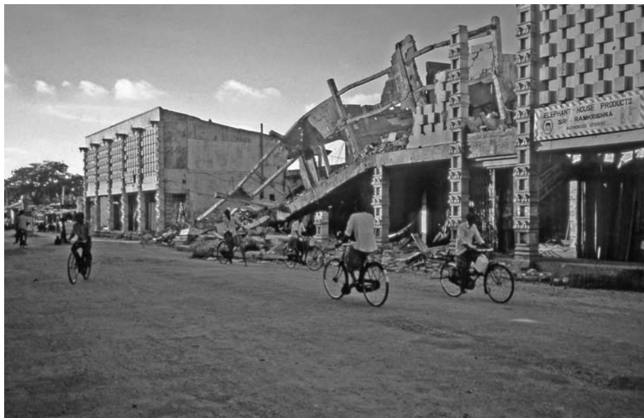
11. Bomb damage in Jaffna (II)
