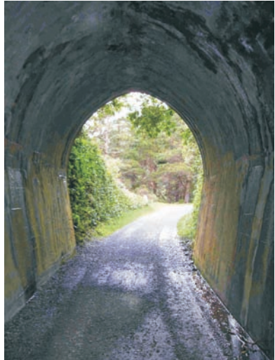
The start of the Rimutaka Incline
