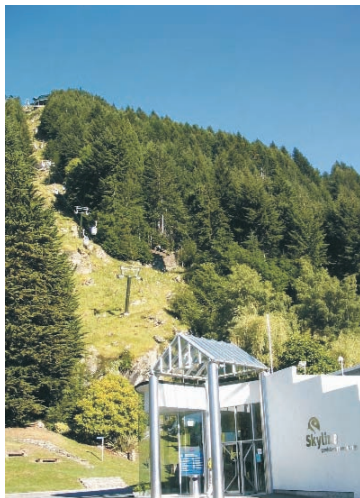
Skyline Gondola base terminal
