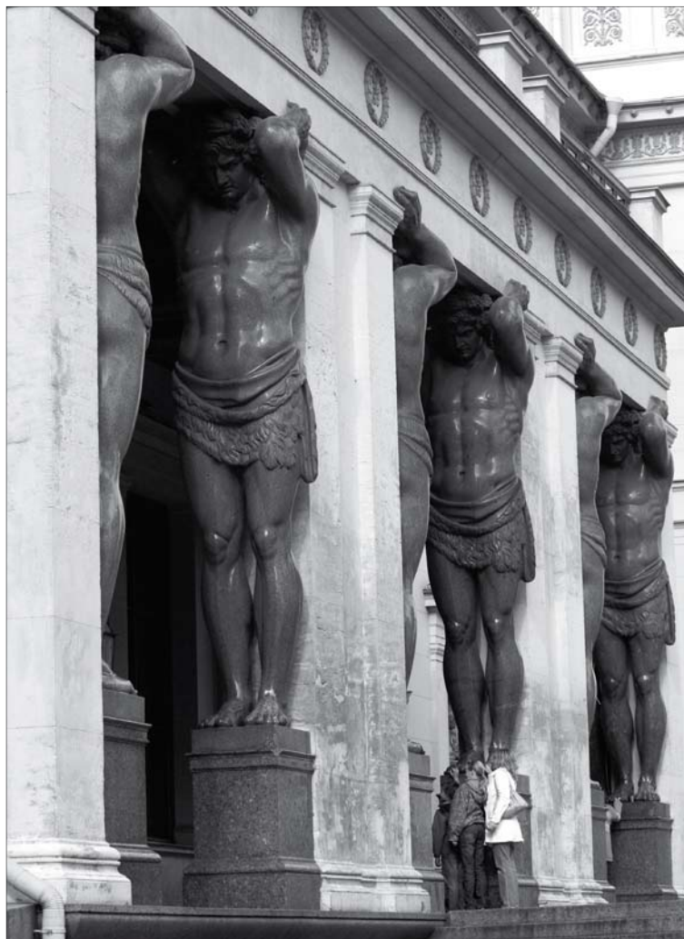
▲ Atlantes supporting the facade
