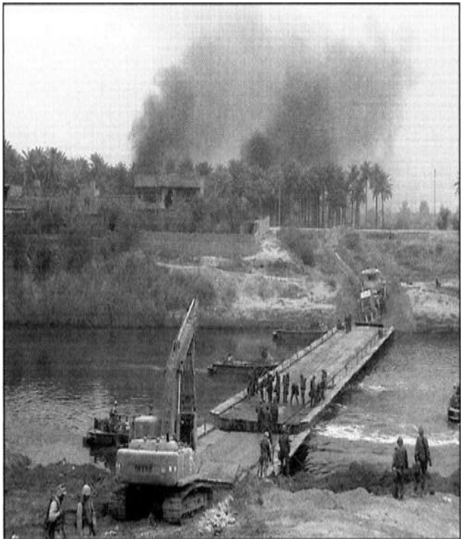
The new bridge we built across the
