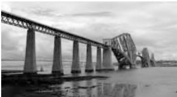
▲ FORTH RAIL BRIDGE
