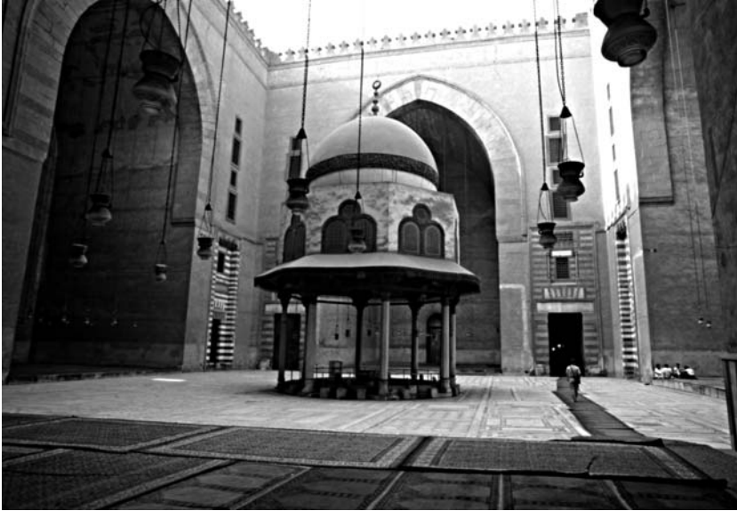
Photo 4.3 The courtyard of the Sultan Ḥasan school in Cairo showing the geometry and spatial order of the centralized open courtyard model.
