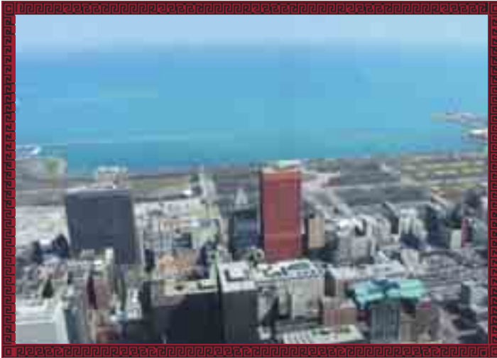
The famous John Hancock Center and the Sears Tower were constructed by a Muslim architect.
