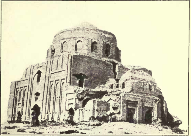
The old ruined Mosque at Tus, Persia, probably dating from the Eleventh Century.
