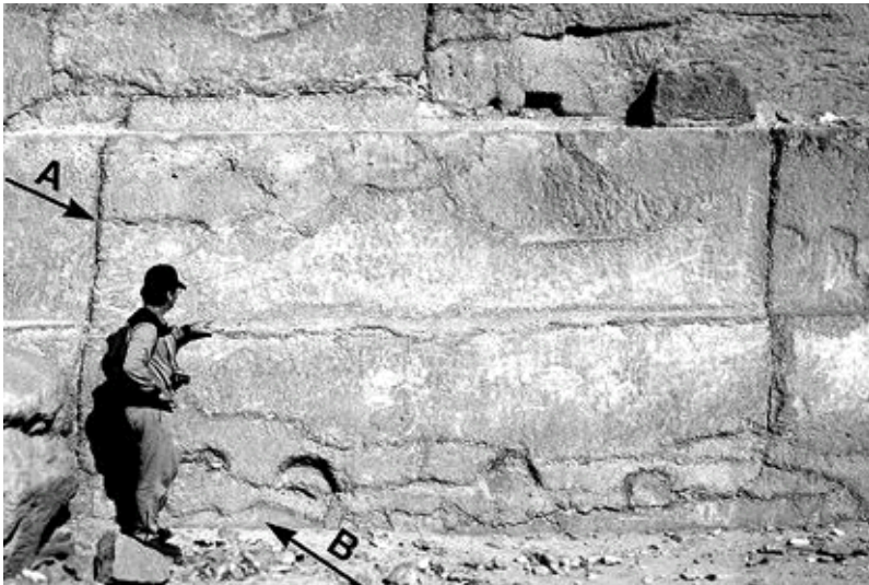
Figure 80: The author examines enormous blocks of the first step on the East Side of Khafra's pyramid. The curved angle joint at (A) suggests stones were cast against bare neighboring stones to produce close fit. (B) Shows thick mortar sealing the bottom of the mold (1984).
