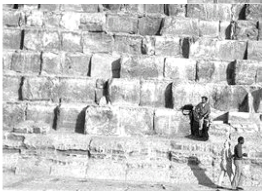
Figure 1c: (bottom) unweathered blocks protected by sand (1984).
