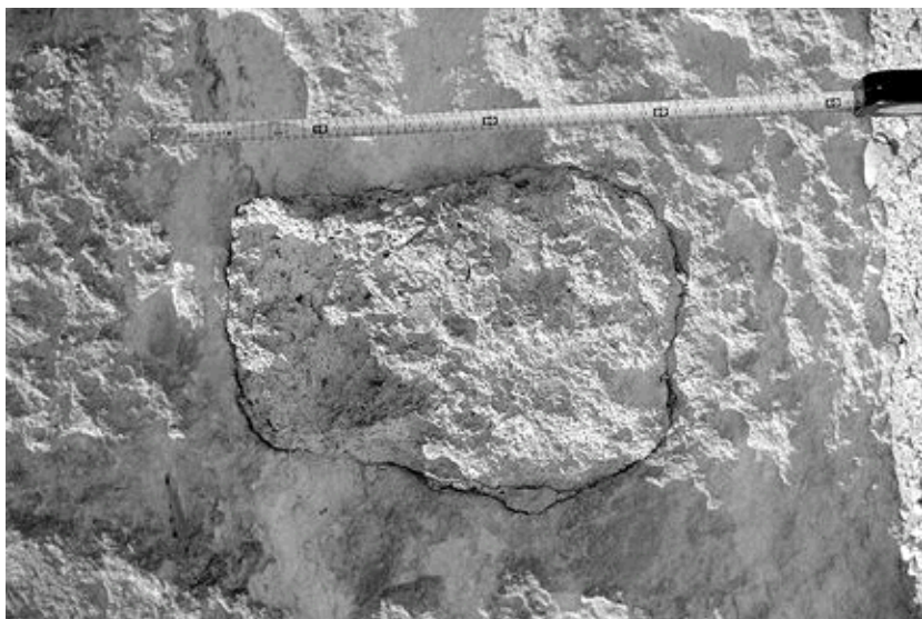
Figure 29: Chunk of stone incorporated into block is visible in Khafra's pyramid (1984).
