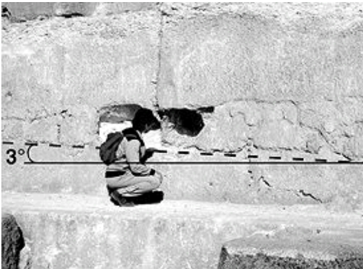
Figure 6b: pyramid blocks above inclined bedrock (dotted line) (1984).
