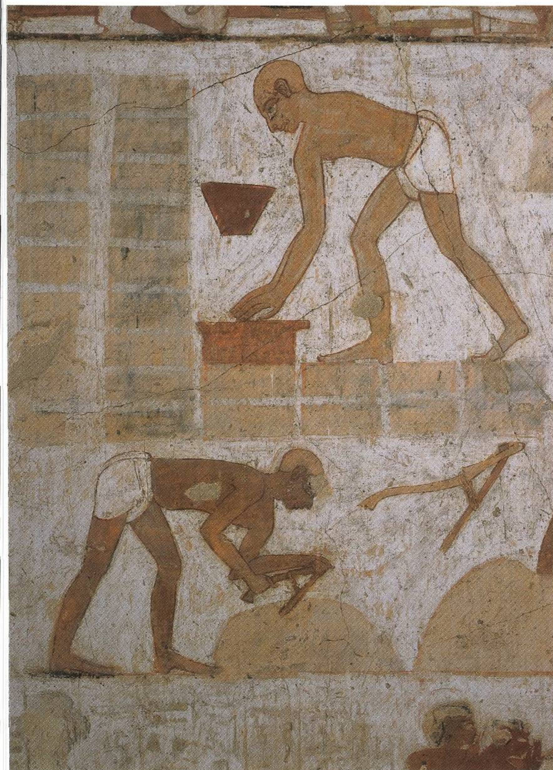
(Above) In this painting from the tomb of Rekhmire at Thebes workmen prepare and lay bricks using a mould. Most of the outlying buildings and walls of Egyptian temples were made of mud-brick.
