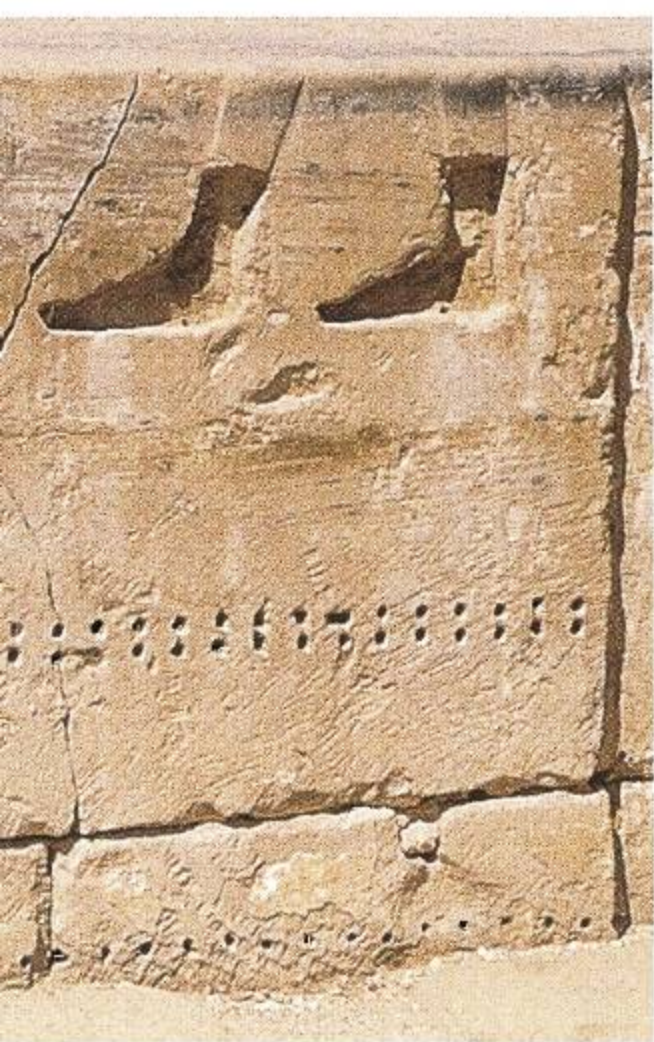
The small holes visible in the side of this doorway at the temple of Ramesses III at Medinet Habu were for metal pins which held hinge panels.
