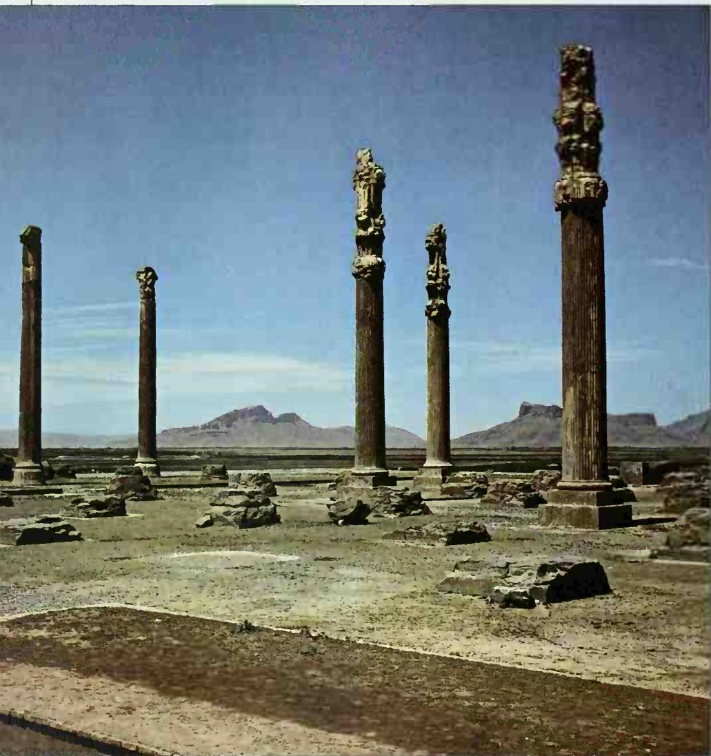
*Five of the surviving slender limestone columns of the apadana rise more than 65 feet. They once held the audience hall's massive wooden roof beams. The two pillars to the left, part of the western portico, were set on fluted, bell-shaped stone bases. The three to the right, resting on simple square blocks, were inside the structure. Originally there were 72 columns in the building; only 13 still stand.*
