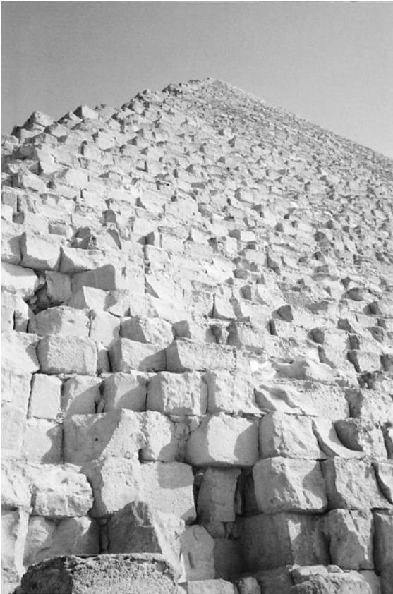
Figure 7.5 Limestone core-blocks in Khufu's pyramid
