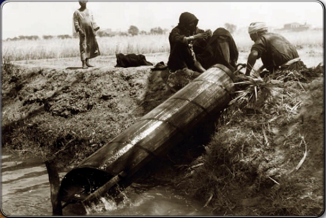
*An Archimedes screw being used to irrigate crops on the Nile delta. The device works as a hydraulic screw to raise water from a lower level.*
