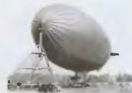
Nonrigid airships have a flexible fabric envelope, from which the load hangs, suspended by ropes.
