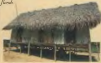
Wooden stilt-house with thatched roof, Malaysia
