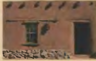
Adobe house built from sun-dried clay bricks, New Mexico, USA
