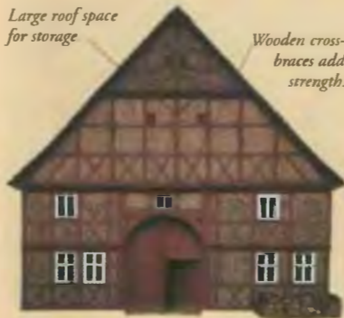
Wood-framed house with brick panels, Germany
