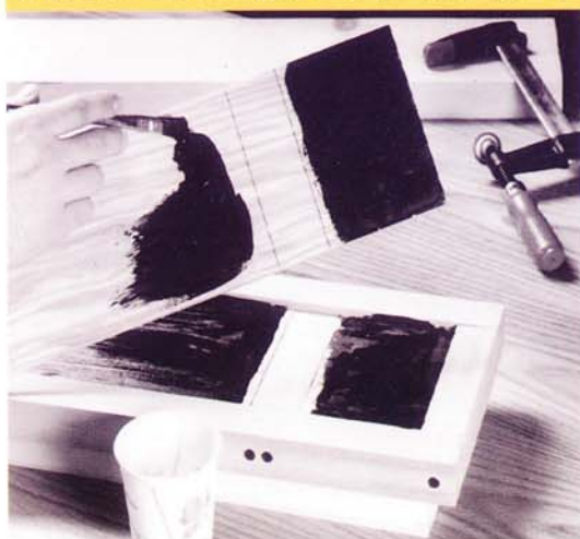
Photo 3 • Apply resorcinol glue to all parts to be laminated. Keep the glue 1/4 inch away from the stake holes to keep squeeze-out to a minimum.
