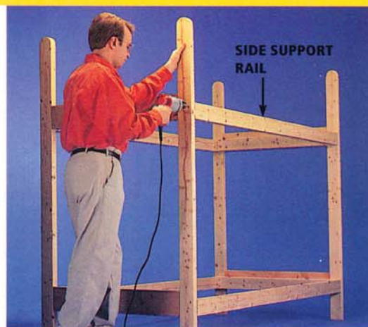
Photo 5 • Attach the long side support rails to the uprights with 3-in. deck screws driven through the corner posts into their ends.
