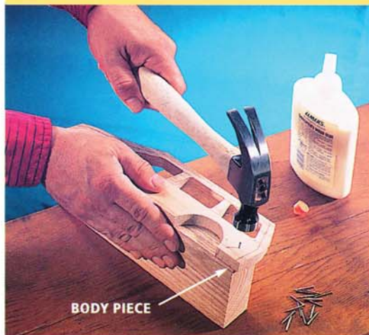
Photo 1 • Fasten the sides with brads to keep them from slipping when you glue them to the angled body piece.
