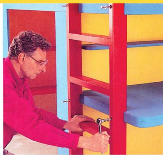
Photo 12 • Reassemble the unit in the bedroom after it's painted, and slide it into the corner. A socket wrench will speed installing the lag screws.
