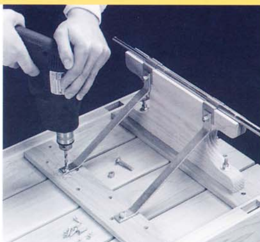
Photo 6 • Use the bolster braces as guides for positioning the inner floorboard cleats. Drill holes through the braces and cleats, and into the mounting floorboards.
