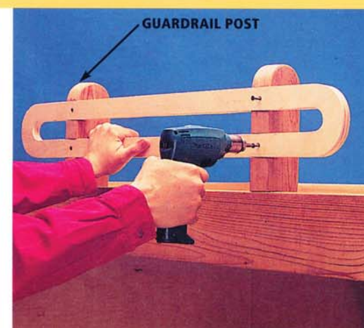
Photo 10 • Make guardrail posts from 2x4's; cut oval rails from 3/4-inch birch plywood, fit them into notches in the posts, and attach with screws.
