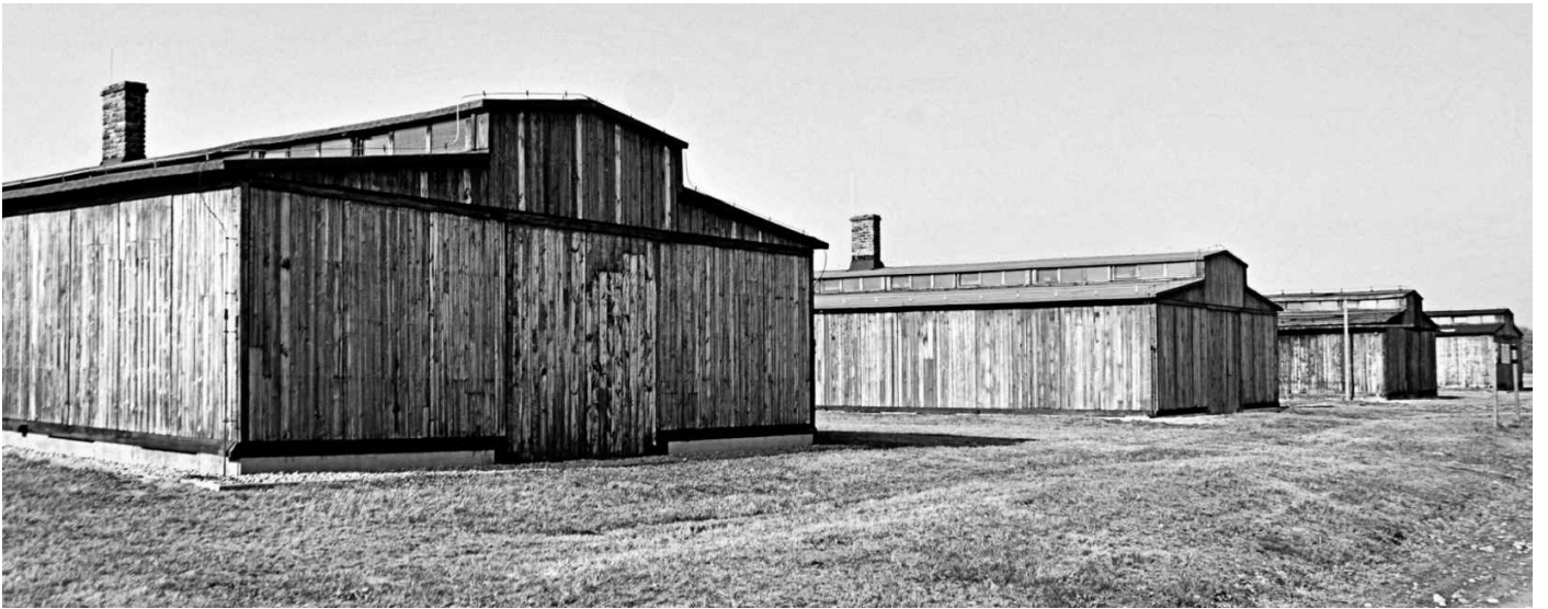
Rebuilt timber barracks remind us of the cramped living conditions.
