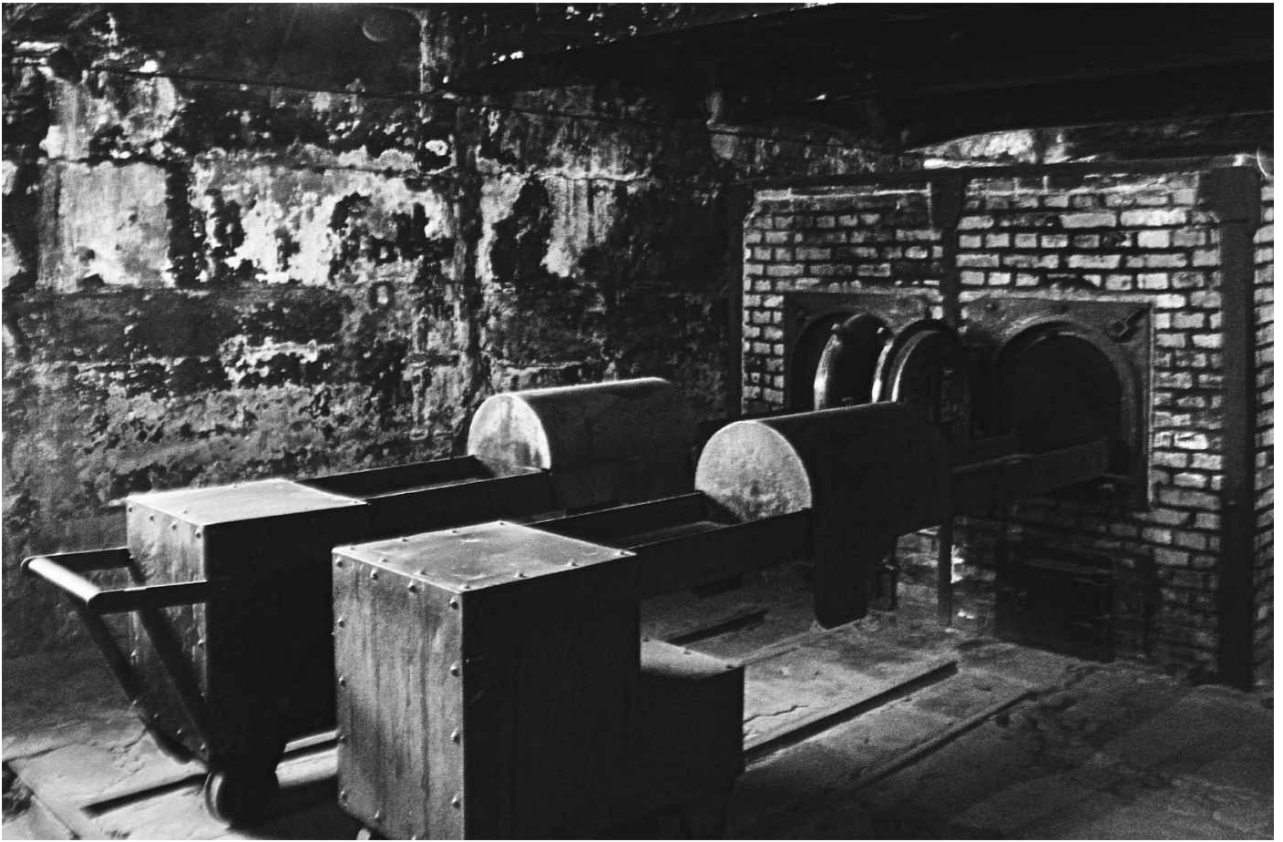
The trollies for pushing corpses into the furnaces inside Crematorium I.
