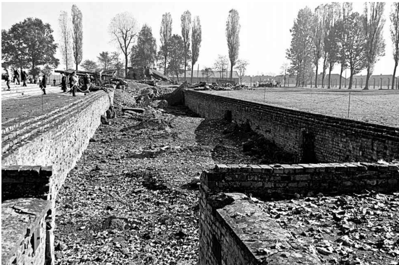
The doomed undressed in this underground changing room before turning right into the gas chamber at the end. The tangle of concrete we can see is all that remains of Crematorium II's furnace hall.
